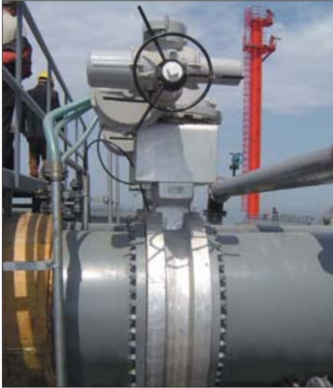
A large Torqseal Triple-Offset Butterfly valve used for crude oil service in Dalian Seaport (China).
